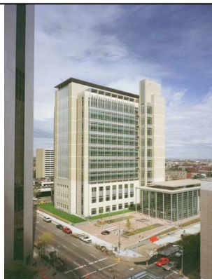
Arraj Courthouse, Denver, CO (Buildings-integrated Photovoltaics)
