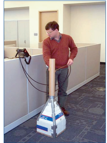
Larry Luskay, Oregon State IAC alumnus, measures air flow rate during the commissioning of an under-floor air distribution system.
