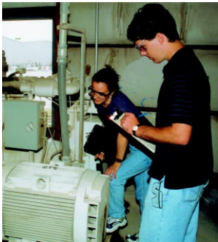
Engineering students, supervised by their professors, record their observations of a compressor operation at a recent IAC assessment.
